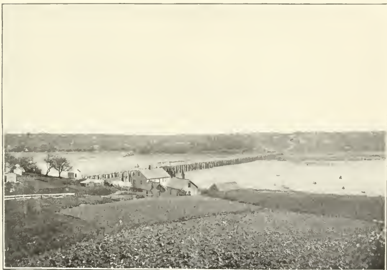
THE LOWER BRIDGE
