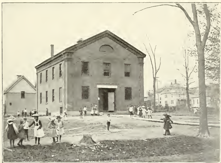
THE ACADEMY. ERECTED 1846. LATER SOUTH PRIMARY SCHOOL
