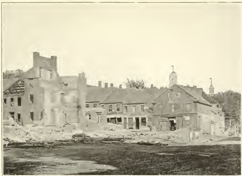
RUINS AMERICAN HOUSE FIRE, 1885
