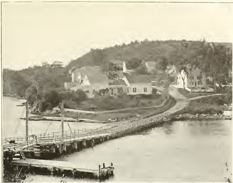
UPPER BRIDGE, PASSAGASSAWAKEAG RIVER
